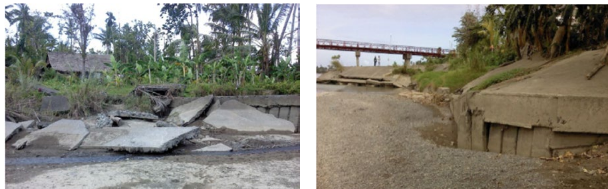
Aklan River. Damage to flood control infrastructure in Libacoo (left). Riprap near Mobo Bridge (right).
