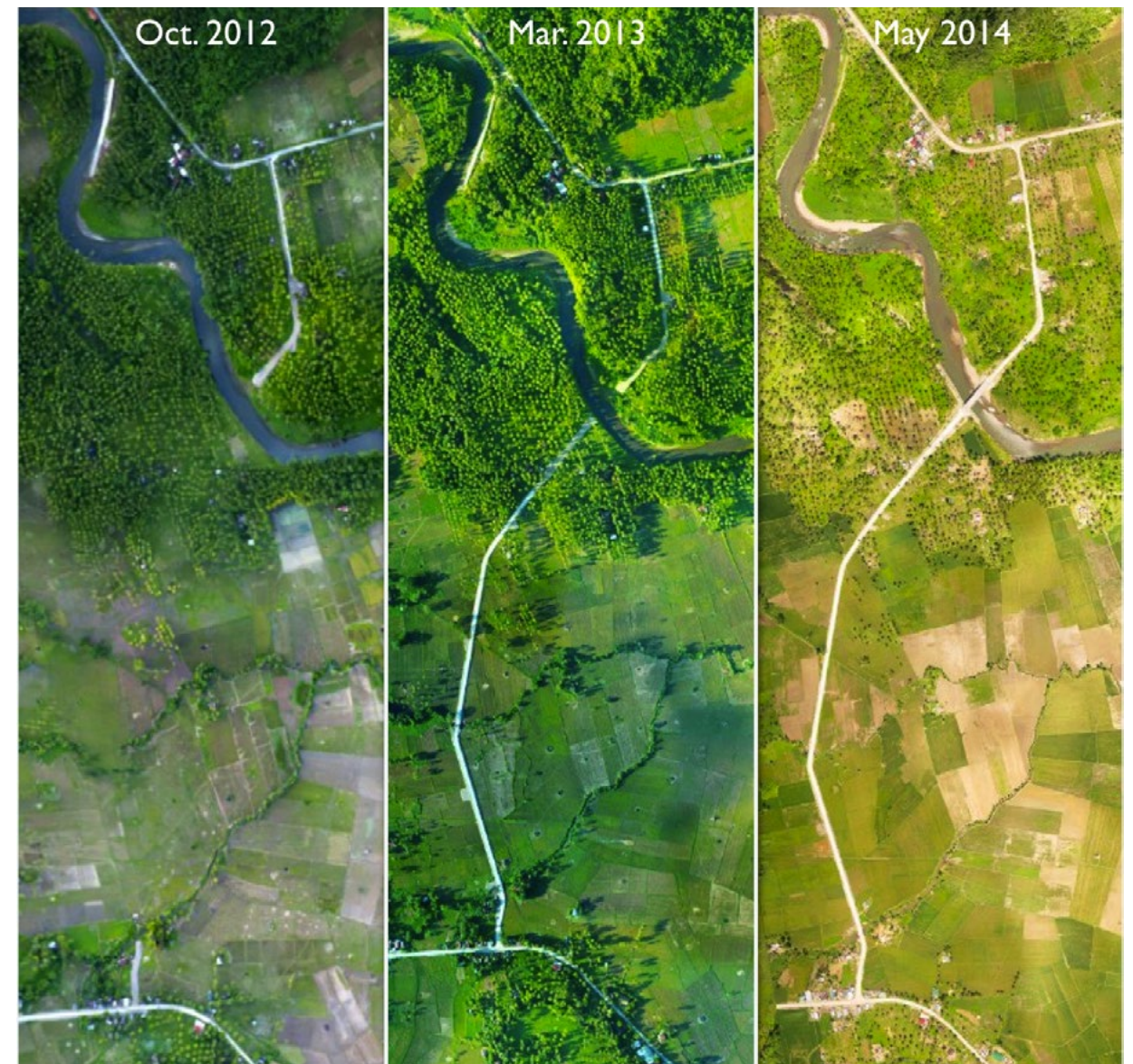
Images taken over the course of a year in the development of a new road and bridge in the municipality of Javier, Leyte. Five months was the span between the two images. In that amount of time, hundreds of meters of road was constructed by the municipal government.
