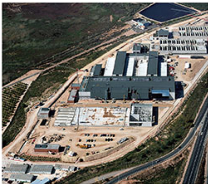
Desalination Plant During Construction
