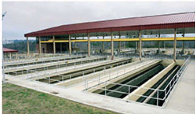
TETRA ® Denite ® at Village Creek WWTW
