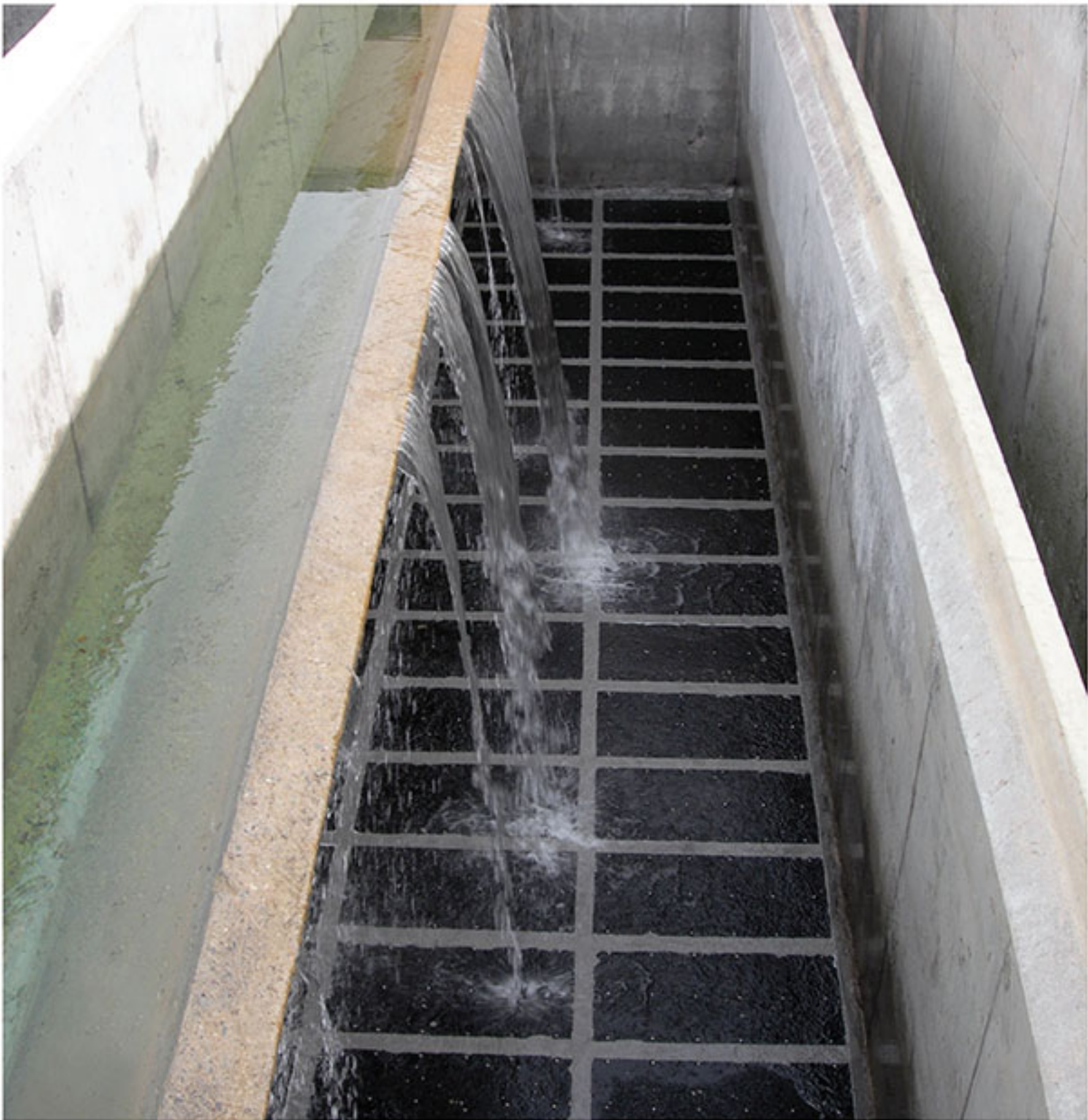
TETRA LP Block™ Dual Parallel Lateral Underdrain Filters
